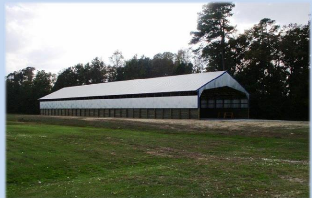
Pictured above is dry litter storage. This structure provides environmentally safe storage of litter and allows for proper timing of litter application to crops. It also stabilizes litter for pathogen and insect control.
