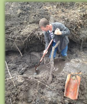
Staff member, Ricky Hayes, digging for old drain tile.
