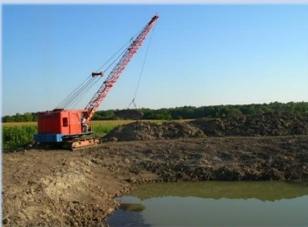
Pictured above is sediment removal to increase water storage for irrigation.
