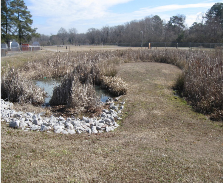
Bio-retention Pond at Wilson Community College
