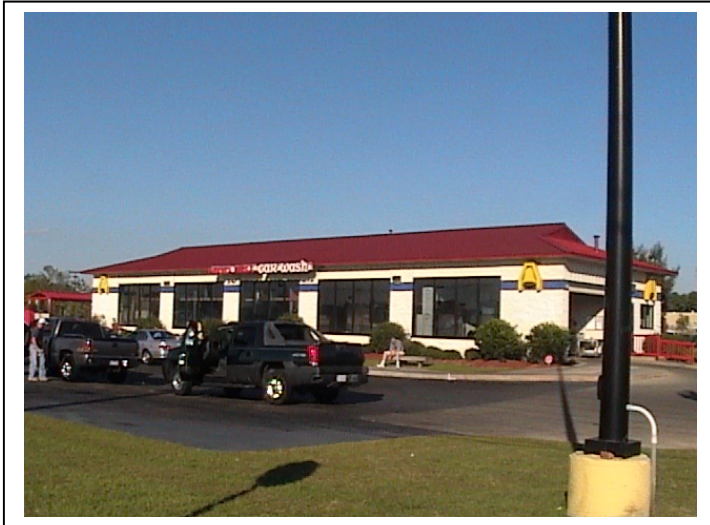
Commercial: Car Wash
