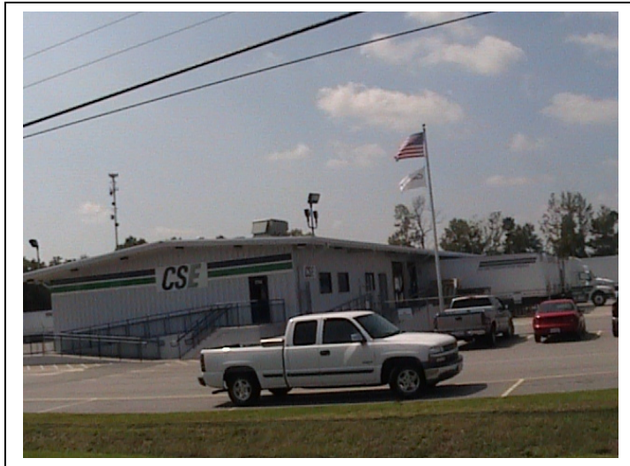
Commercial: Truck Terminal
